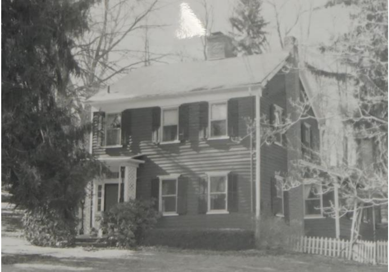
Photograph 45 Belden Hill Road. View northeast.
