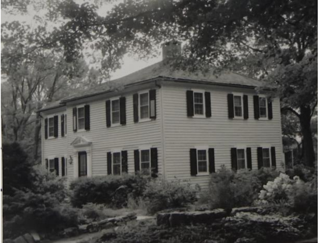
Photograph 923 Ridgefield Road View Northeast
