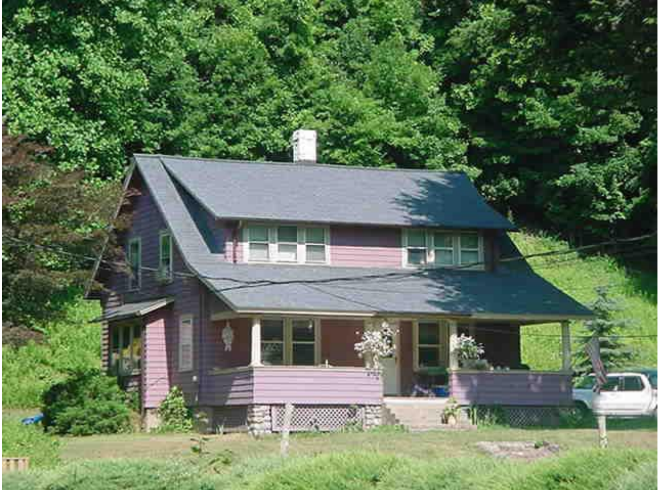
Photograph 763 Danbury Road. View East.
